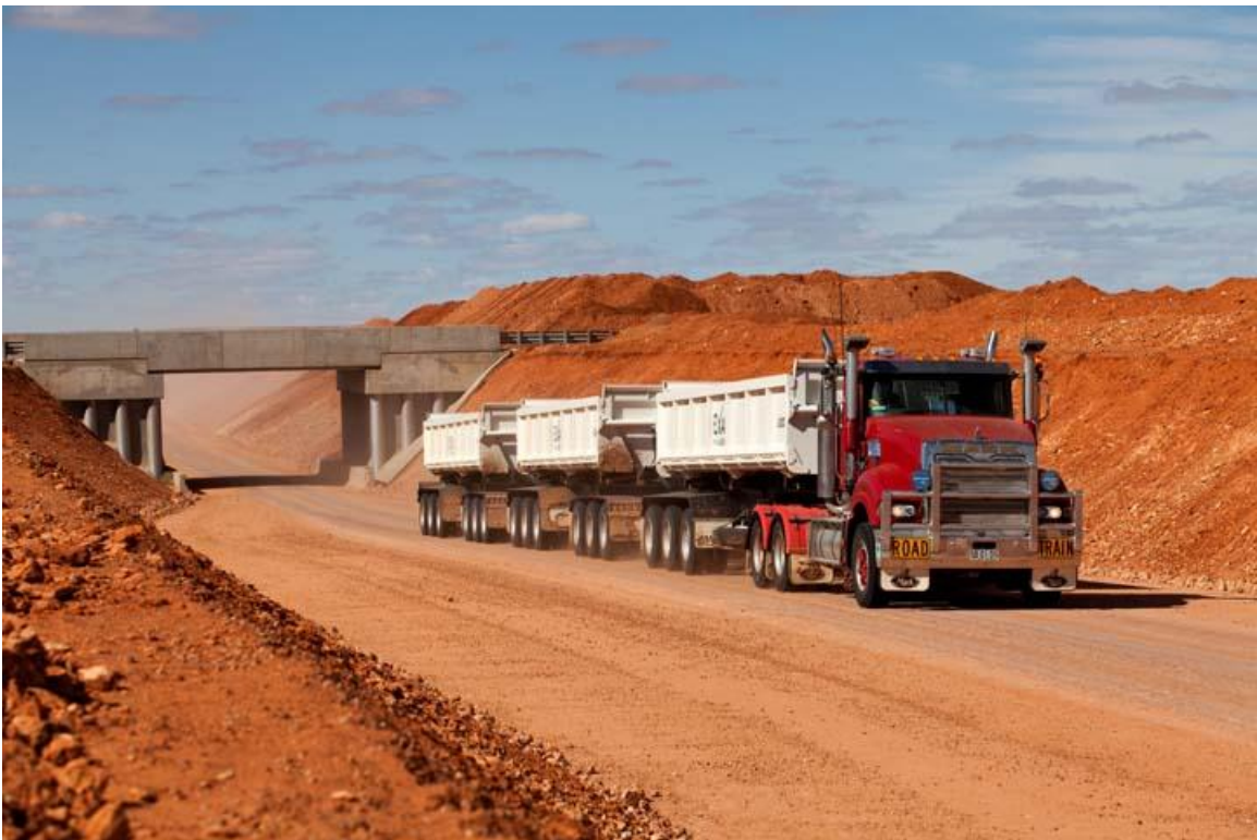
Photo 2: Roadtrain travelling to Rankin Dam (rail siding) after passing through Stuart Highway Underpass
